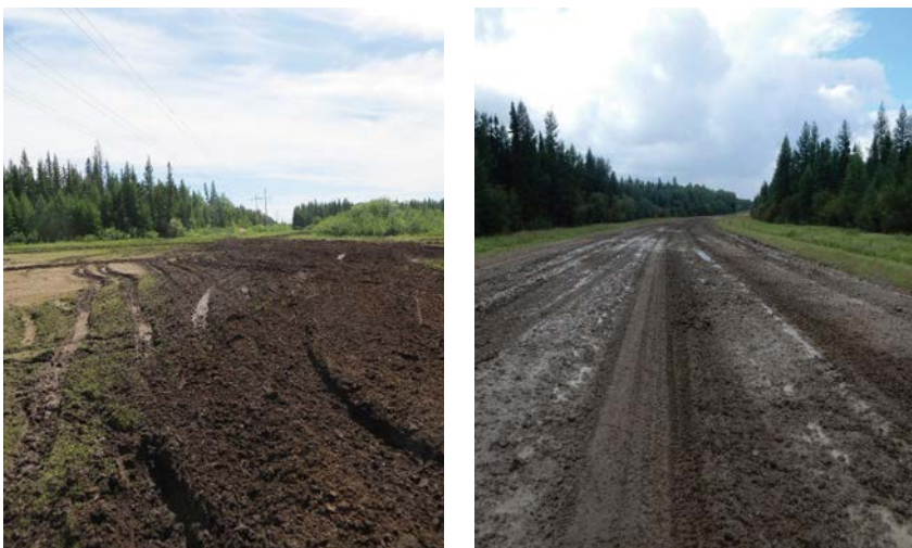
FIGURE 14. Examples of soil compaction and rutting from off road vehicles along powerline right-of-way near Grande Prairie, Alberta (left) and from highway vehicles on access road near Wabasca, Alberta (right).
