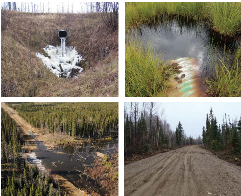
FIGURE 10. Example of wetland road challenges clockwise from top left: perched culvert, sunken culvert, blocked flow, and road compaction.
