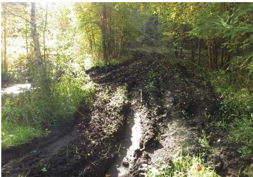
FIGURE 12. Example of soil rutting and compaction
