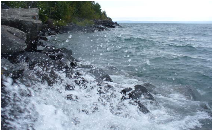
Rip Rap at Silver Harbour Conservation Area
