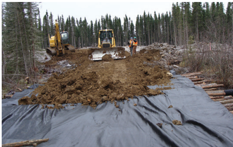
Geotextile used as a separation layer.
