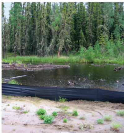
Example of poorly installed sediment fencing (left) and well installed sediment fencing (right) to control erosion and sedimentation.
