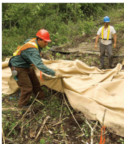
Use of biodegradable geotextile is suitable for temporary crossings.
