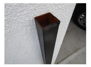
There is minor corrosion on some areas of the metal fencing and some areas are not completely painted.
