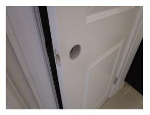
The door margin is inconsistent at the downstairs bedroom door and the third floor hall closet door. This condition is causing these doors to be hinge bound. These doors should be adjusted so that the margins are 1/8 to 3/16 of an inch consistently.
