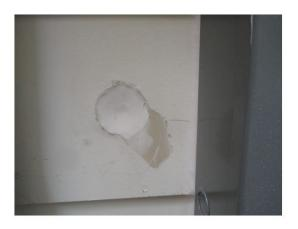
Some of the corners of the exterior siding are damaged in several areas and there is a damaged piece of exterior trim at the rear southwest corner of the home.
