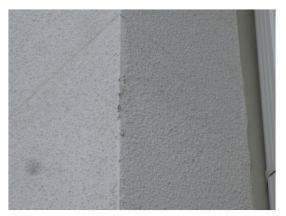
The exterior siding has been installed notably not level on the front of the home at the fourth floor deck area.
