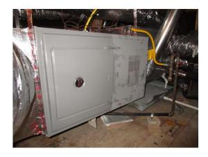
**Comments:** The furnace was not operational as the gas supply to the equipment at the time of the inspection.
