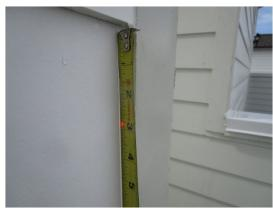
There are large gaps under the stucco walls at the front of the garage where the bottom wall plates are not complete and the walls are cantilevered off the foundation leaving the structure exposed.
