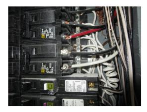
An inhibitor paste has not been applied to the main aluminum wires. The surface of aluminum can oxidize when it is exposed to air resulting in a poor connection.
