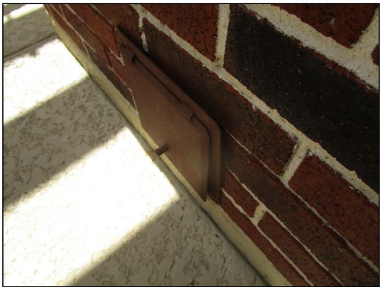
The ash dump door on the exterior is loose.
