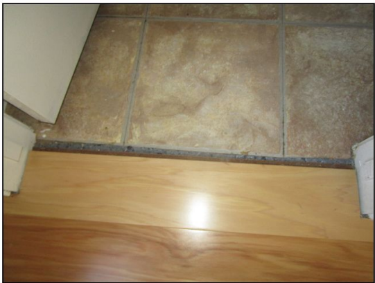
There was evidence of water penetration (water stain) on the ceiling of the upstairs rear northeast bedroom. This area was dry when tested. Leaks can cause hidden or concealed damage. All damaged elements should be repaired or replaced. The reason for the water penetration is unknown. This area should be monitored, especially during heavy rain, to determine if the leak is active.
