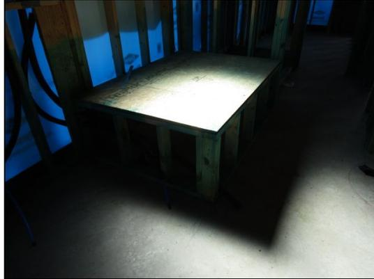
It is necessary that there be an inspection port provided for the whirlpool bathtub so that it is possible to check for leaks and have access to the pump motor when the home is complete. There was no access to this area at the time of the inspection. This does not comply with National Electric Code (Ref. NEC 680-72) Accessibility. "Hydro massage bathtub electrical equipment shall be accessible without damaging the building structure or building finish.
