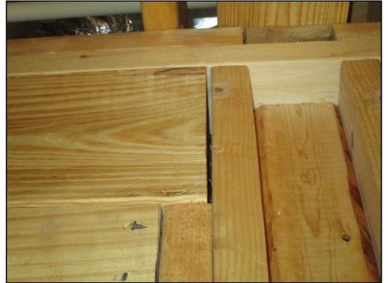
A protection plate (nail guard) needs to be installed at the bottom plate in the back of the media room to prevent nails/screws from puncturing the HVAC duct.
