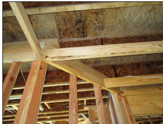
Several nails from the second floor sub flooring in the study and in the rear west side bedroom have missed the ceiling joists. It is recommended that these nails be removed as they may cause squeaks in the upstairs floor to develop in the future.
