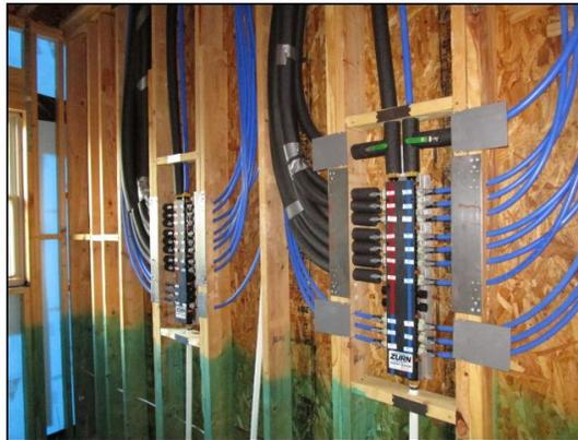
**Comments:** There was no water supply to the home as is necessary in order to check for possible leaks before the installation of the sheetrock and insulation.
