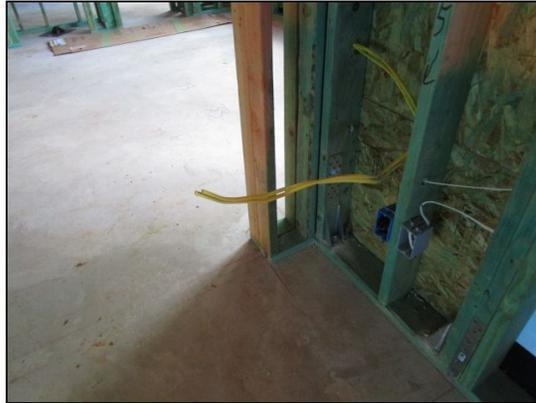
The rough in wiring for the outlet in the communication box has not been installed in the upstairs front middle bedroom closet.
