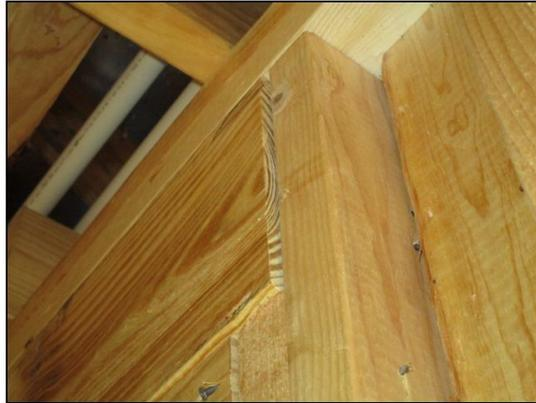
It is necessary to shim/fill the gaps between the wall framing at the supporting headers.
