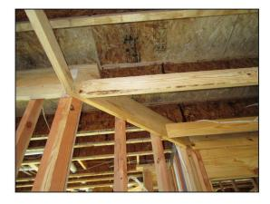
Several nails from the second floor sub flooring in the study and in the rear west side bedroom have missed the ceiling joists. It is recommended that these nails be removed as they may cause squeaks in the upstairs floor to develop in the future.
