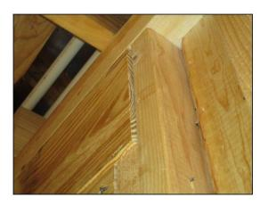
It is necessary to shim/fill the gaps between the wall framing at the supporting headers.
