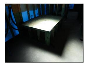
It is necessary that there be an inspection port provided for the whirlpool bathtub so that it is possible to check for leaks and have access to the pump motor when the home is complete. There was no access to this area at the time of the inspection. This does not comply with National Electric Code (Ref. NEC 680-72) Accessibility. "Hydro massage bathtub electrical equipment shall be accessible without damaging the building structure or building finish.
