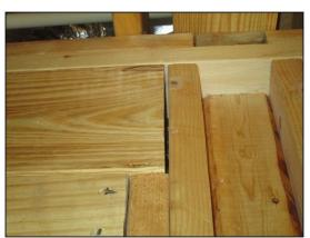
A protection plate (nail guard) needs to be installed at the bottom plate in the back of the media room to prevent nails/screws from puncturing the HVAC duct.
