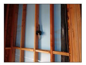
There are electrical wires that are not inside of an outlet or junction box on the rear wall of the living room.
