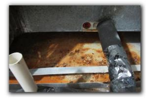
The main drain line from the second floor zone coil box is not fully insulated. This line should be insulated for at least 10' from the coil box unit. This condition causes the lines to sweat and may also cause water damage because they are located in the attic area. Applying foam tubes and taping them will remedy this condition.
