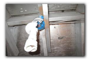
Wires were improperly spliced terminated at the light fixture in the attic at the water heater/elevator equipment area. Wire ends or splices should be in junction boxes that are properly mounted. This condition is considered an electrocution/fire concern and should be serviced by a licensed electrician.
