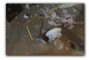
Several of the electrical outlets in the home are loose and need to be secured to avoid possible loose connections/electric shorts.
