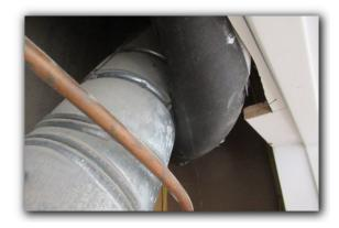
There are no condensate drip legs/sediment traps installed on both of the furnace gas supply lines as is now required.
