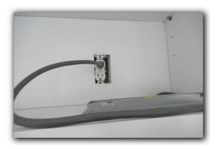
A polarity problem was detected as the hot and neutral wires appear to be reversed at the outlet inside the first level storage closet in the back of the home. Outlets are checked using a circuit tester. As fixing one outlet may cause other outlets down the line to have problems, I recommend that the system in this/these areas be serviced by a licensed electrician.
