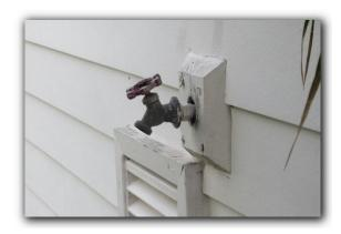
It is recommended that all of the exterior water lines be insulated from the weather in order to prevent freezing.
