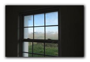
Window screens were not installed. Screens are mentioned in this part of the report as they are a specific item in the T.R.E.C. Guidelines. All windows that have channels for screens should have them installed.
