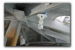
The light fixture in the master bathroom shower area is not flush with the ceiling.
