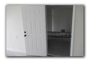
The door hardware is incomplete at the exterior closet ground floor door.
