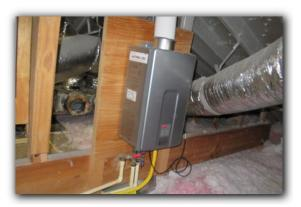
**Comments:** There was no condensate drip leg/sediment trap installed on the water heater gas supply line as is now required.
