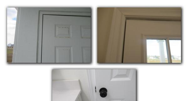
There is no self closing device installed on the door from the house to the garage.
