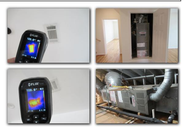
**Comments:** The second floor zone furnace flue pipe is in contact with the AC refrigerant line insulation. Gas appliance flue pipes must have a minimum of 1" clearance from any combustible materials.
