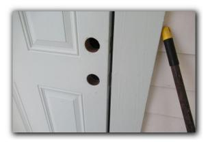
The exterior trim has been water damaged and there is corrosion at the exterior storage closet door off the third level deck. All damaged elements should be repaired/replaced.
