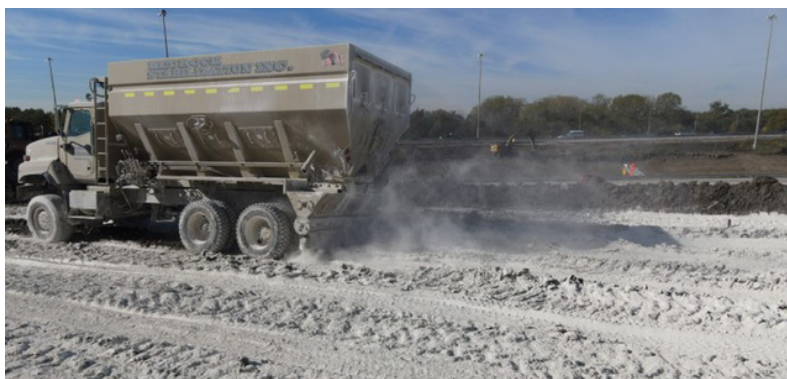
The contractor, Bedrock Stabilization, laying the pulverized quicklime
