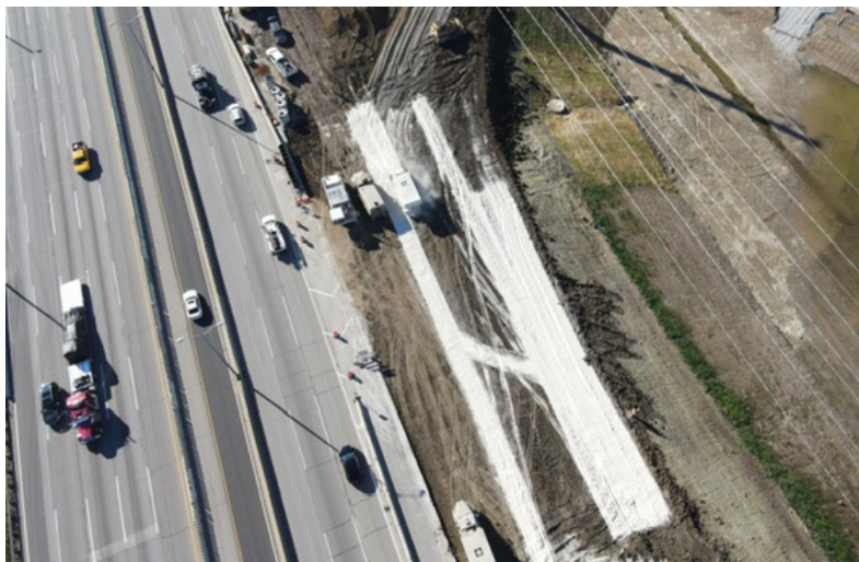
Aerial view of the I-294 job
