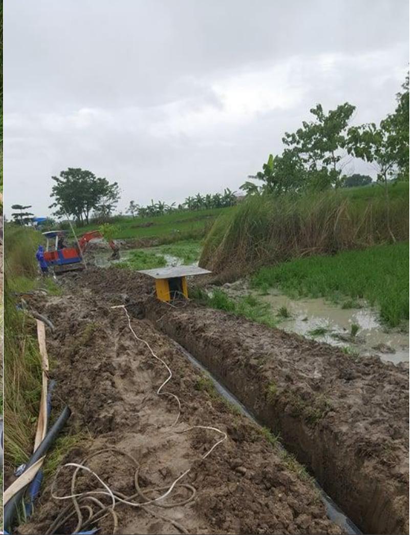
800 Meters pipe laying project Total of 90 pcs 8x9M S17 Black HDPE Pipe Total Butt Fusion: 89 Working weather condition: During typhoon Fabian
