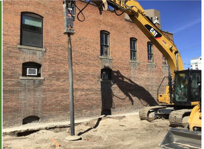
According to the measured values, the maximum ground vibrations for the three Aggregate Piers closest to the building was 0.193 in/s, 0.195 in/s, and 0.160 in/s. These vibrations occurred at a frequency of roughly 64 Hz.
