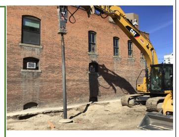
According to the measured values, the maximum ground vibrations for the three Aggregate Piers closest to the building was 0.193 in/s, 0.195 in/s, and 0.160 in/s. These vibrations occurred at a frequency of roughly 64 Hz.
