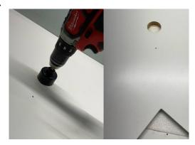
Using a hole saw (1 ¾"-2"), cut a hole at point B.
