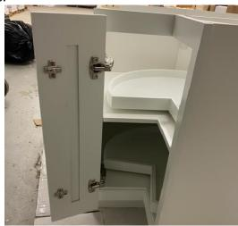
Mount hinges to face frame. (hinges can be mounted to either side of the frame.) Then attach doors to the hinges.
