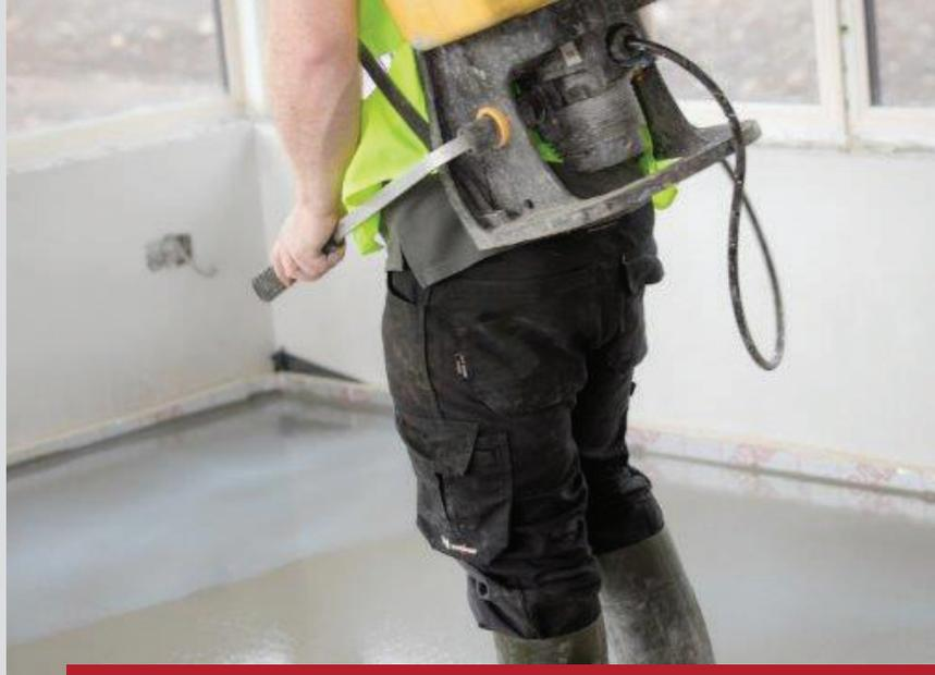
Cemfloor EC is a white, spray-applied high performance compound designed to ensure the full curing of Cemfloor liquid screed. Once applied it functions by retaining the hydration moisture at the surface of the freshly placed liquid screed during the initial 12 to 24 hours. It is formulated to prevent early evaporation of the gauging water and provides an economical and highly efficient method of retaining moisture at the surface during the early stages of hydration.
