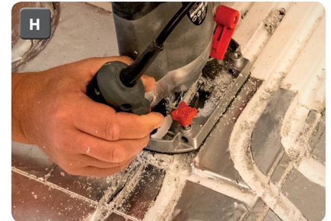
Using a router with bit set to 17mm depth gentle cut the new channel following the marker pen layout **(H)**. Ensure the channel is clear and free from debris, if required the channel can be lined with aluminium tape. Lining with aluminium tape is not required in areas with highly concentrated/close floor heating pipes.
