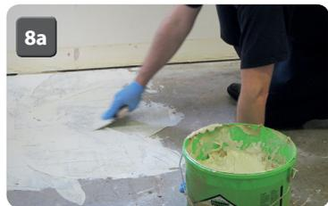
**8a** Starting with a few square meters at a time apply Mapei Ultrabond ECO 380 to the substrate using a 2mm (A2) tooth comb spreader (8a). Do not use Mapei Ultrabond ECO 380 as a filler to level out gaps, cracks or uneven substrates as this will greatly reduce the coverage achieved and increase drying times. Any uneven screed or concrete floors should be levelled with a renovation screed first.
