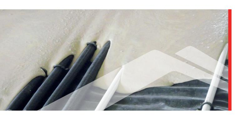
Gypsol Rapide is a unique and highly innovative faster drying screed which uses high quality Gypsol anhydrite, specially graded sands and selected additives to create a free flowing self-compacting and self-smoothing floor screed which dries in a fraction of the time taken for more traditional anhydrite or cementitious screeds. This allows the user to install floor coverings in significantly less time than for competing screed systems.
