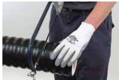
(2) Cut the casing pipe with a saw.
