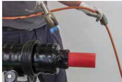
(8) Fit the Heat-Shrink End Cap (see section 5.4.1).
