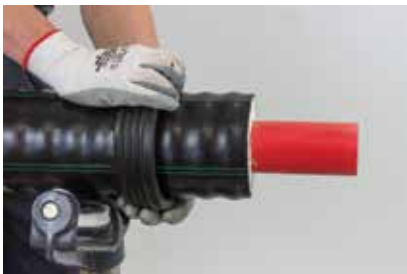
(7) Install the wall sealing ring.
