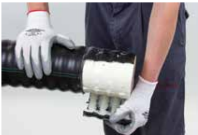
(4) Peel off the casing.
