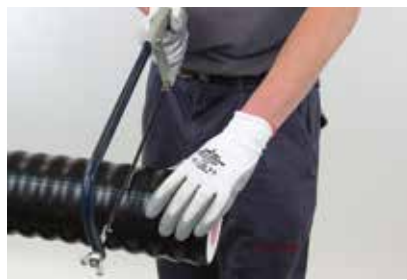
(2) Cut the casing pipe with a saw.
