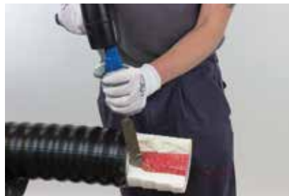
(5) Cut back and remove the insulation along the length (see table for dimension L).
