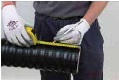
(1) Mark the distance L plus 10mm from the end of the pipe.
