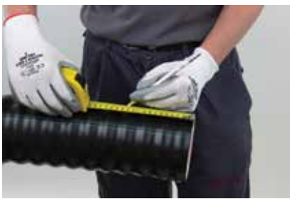
(1) Mark the distance plus 10mm from the end of the pipe.
