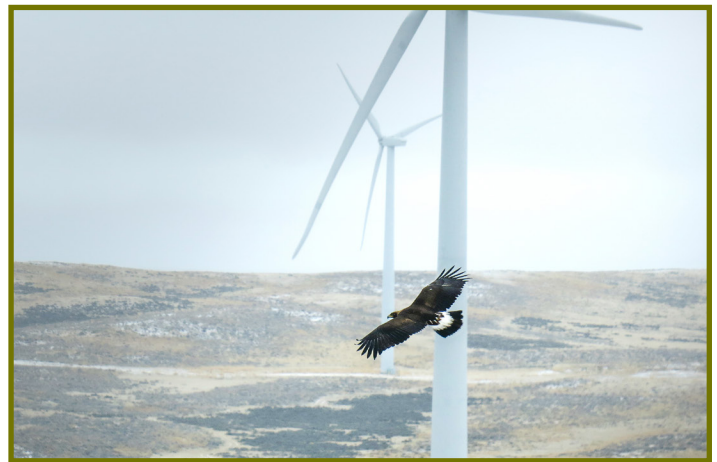
Wind turbines pose a threat to Golden Eagles from direct injury and mortality, and from habitat loss and modification during and following construction. Taylor Berge
