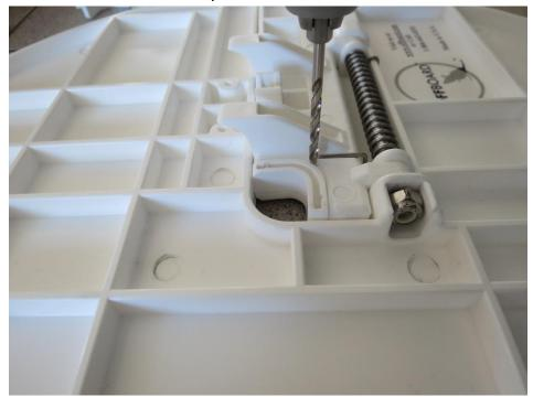
3) Using a 1/8 drill bit and the notch as a starting point, drill a hole vertically through the insert and the door making sure the hole goes through to the other side.
