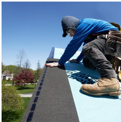
Installs at eave and rake edges to help prevent shingle blow-off.
