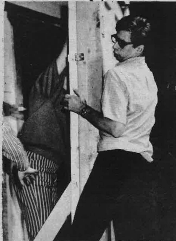
Mike Shaw lends a hand to set construction by bracing a flat.
