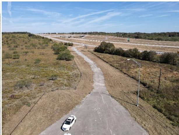
View looking back at entrance gate & HWY 130
