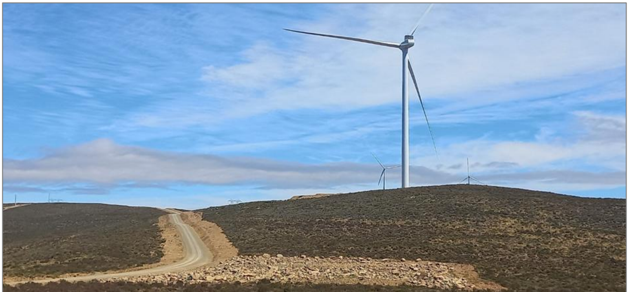
Figure 4: Crusher located at Road 5, ripped and levelled
