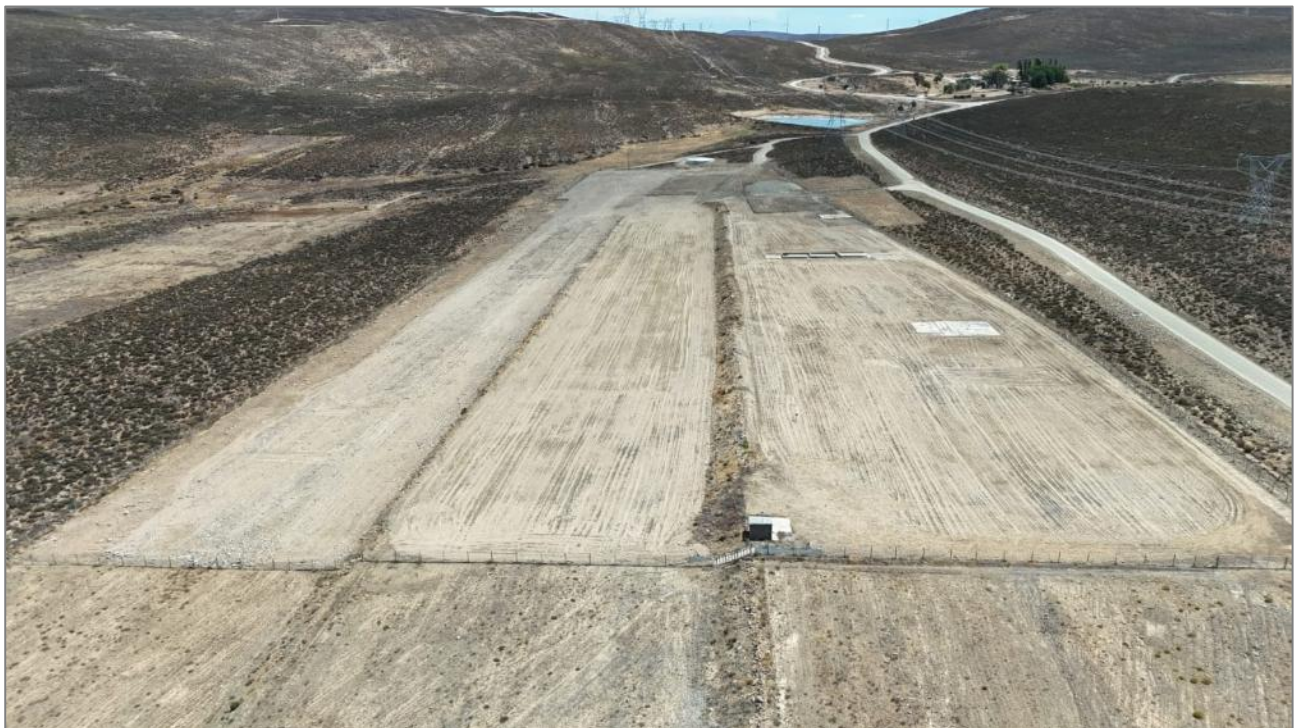
Figure 8: Aerial view of main site camp
