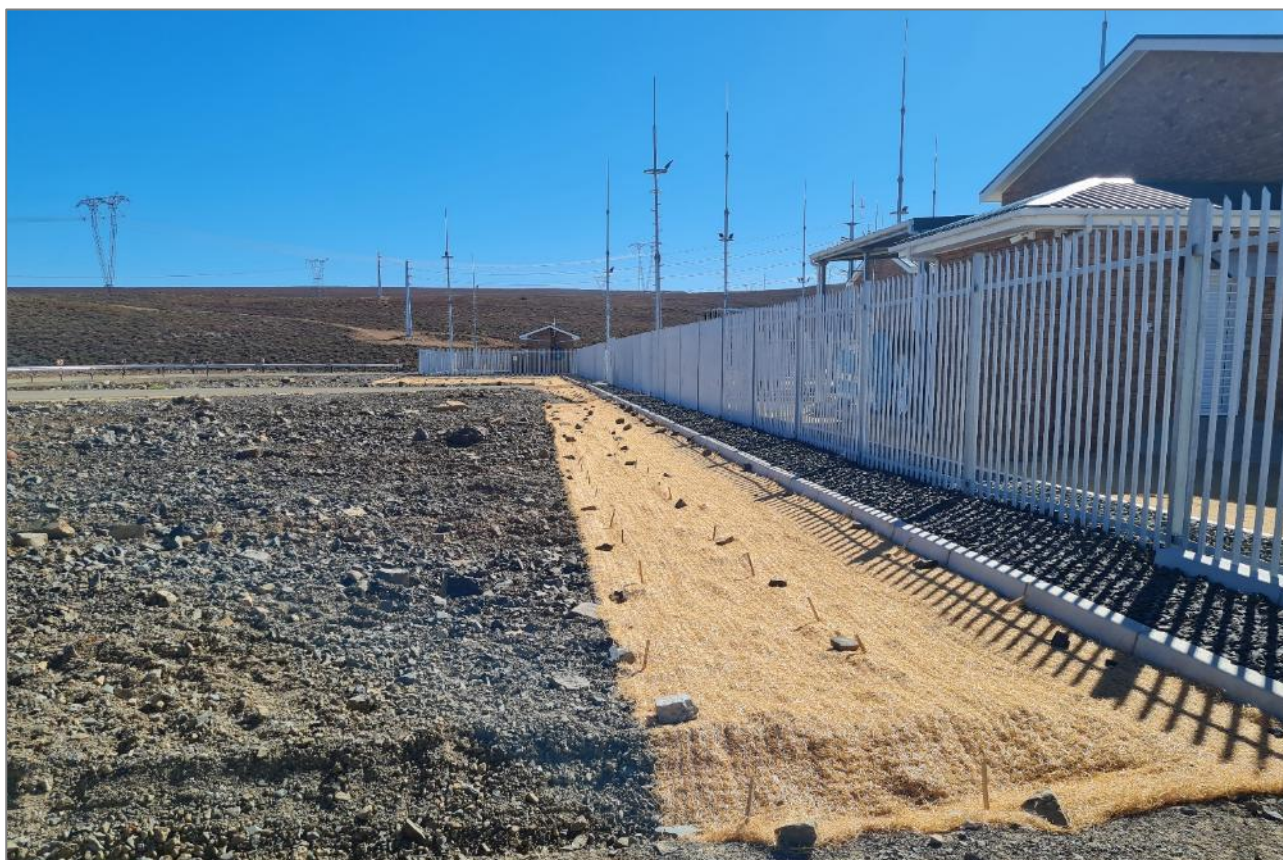
Figure 1: Completed Brandvalley Substation with erosion mitigation netting in place.
