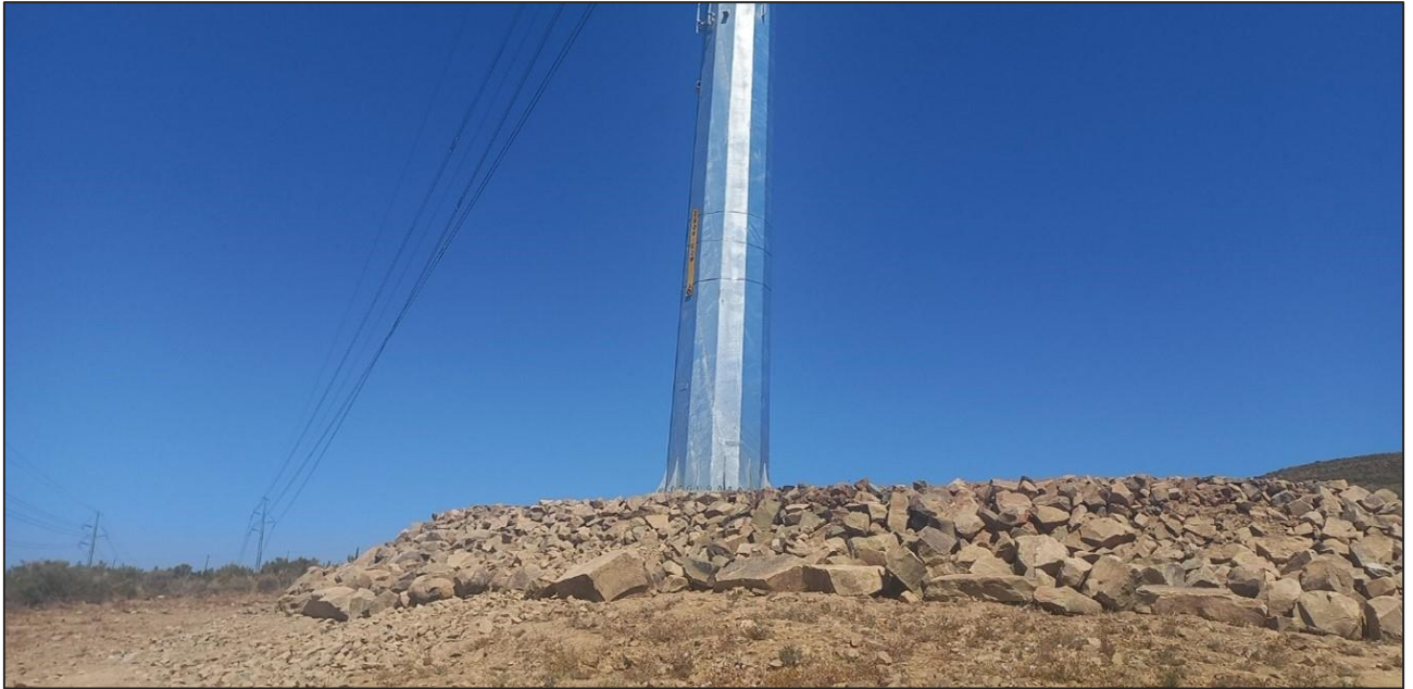
Figure 3: Stone pitching
