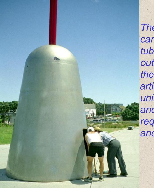
The Wind Wand is a carbon fiber reinforced tube, cylindrical on the outside and tapered on the inside, to meet the artist's demand for a uniform outside diameter and the engineering requirement for strength and weight optimization.
