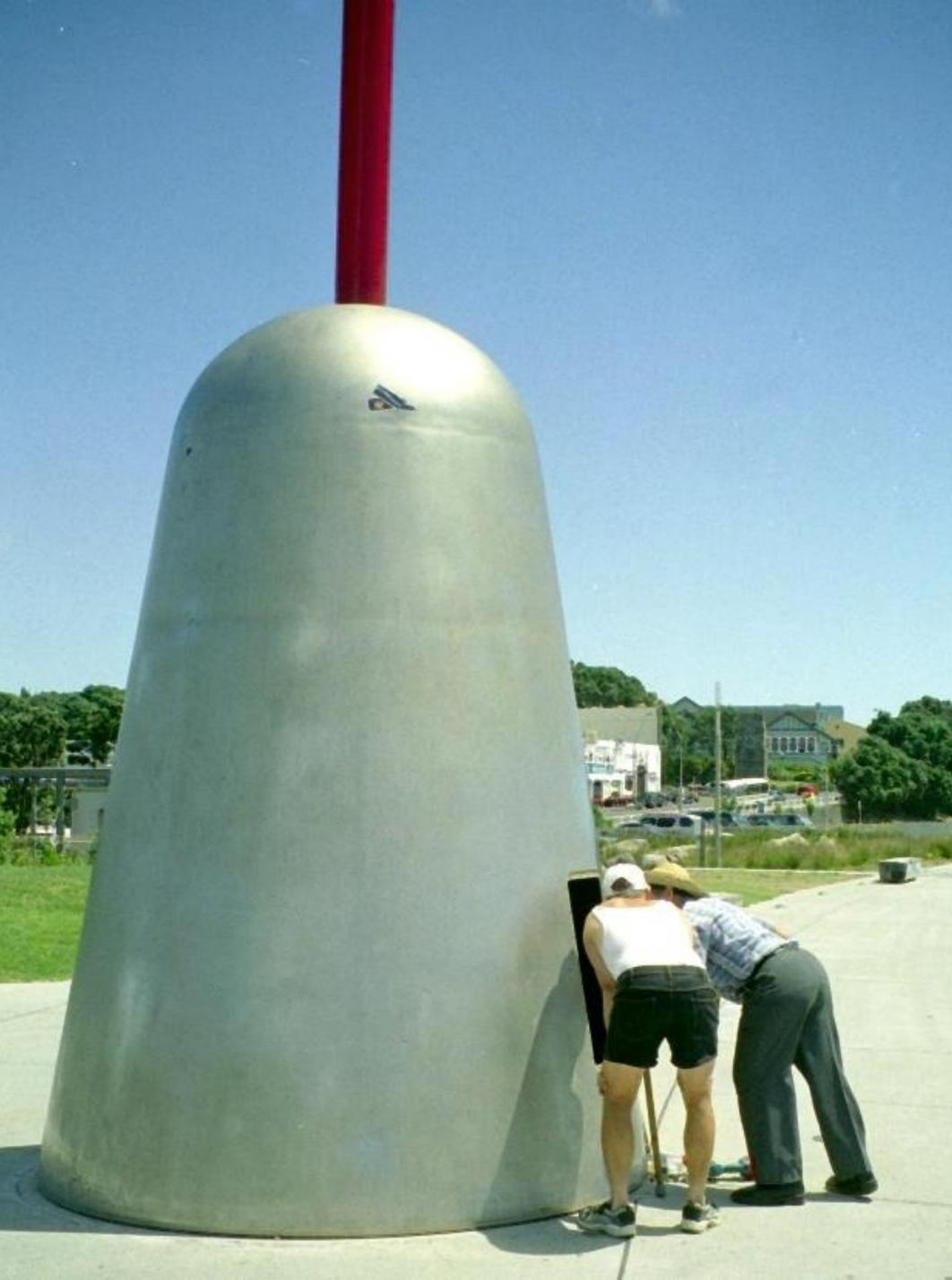
*The Wind Wand is a carbon fiber reinforced tube, cylindrical on the outside and tapered on the inside, to meet the artist's demand for a uniform outside diameter and the engineering requirement for strength and weight optimization.*
