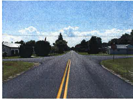
Old Mill Rd EB approach to Railway Rd
