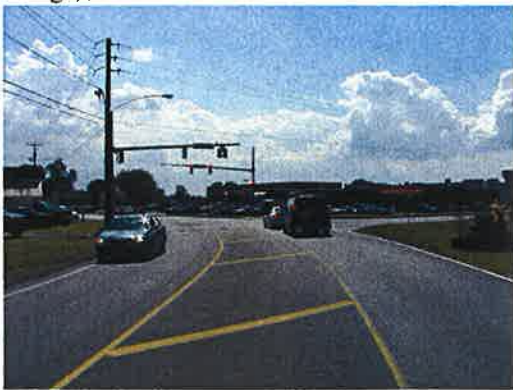
Del Rte 26 EB approach to Del Rte 17
