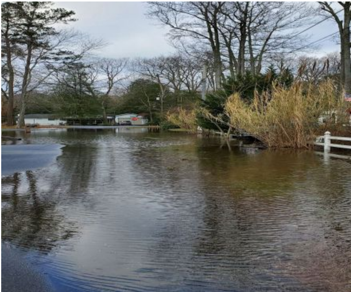
Impassable Street in Banks Acres, Pine Street Looking towards Railway Road.
