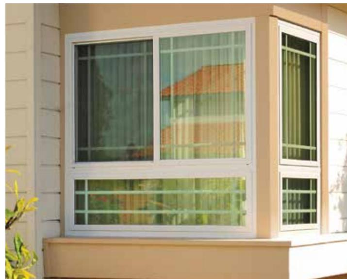
▲ Madeira windows and doors can be mullered together for virtually unlimited configurations.
