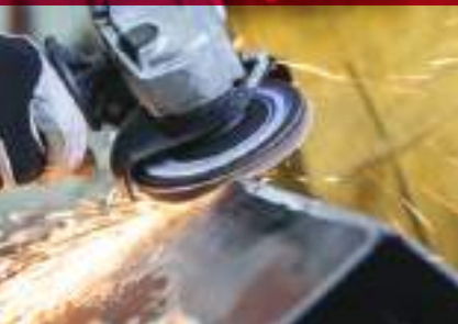
Blending and finishing a weld with a Big Cat flap disc.
