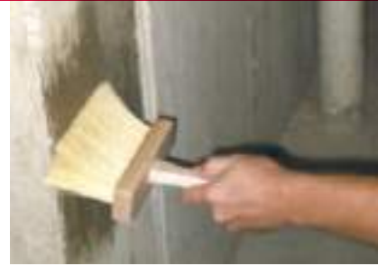
Applying waterproofing material with a masonry brush.
