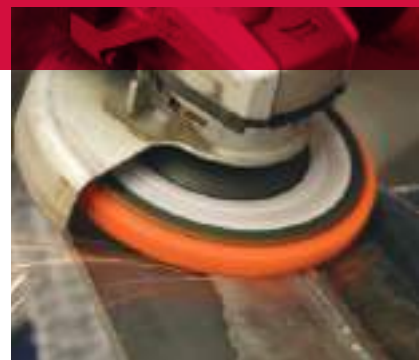
Weld cleaning with a strip disc.
