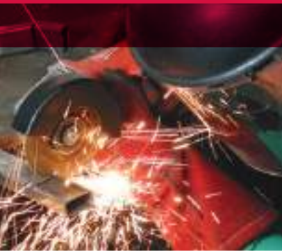
UltraCut wheel making precision cuts on steel tube stock.
