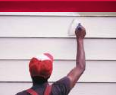
Applying paint to clap board siding.
