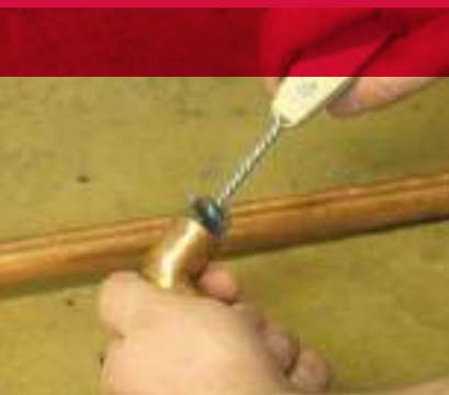
Cleaning the inside of a copper fitting prior to soldering.
