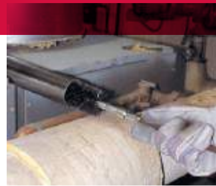
Cleaning boiler pipes with a flue brush.
