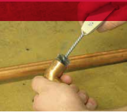
Cleaning the inside of a copper fitting prior to soldering.
