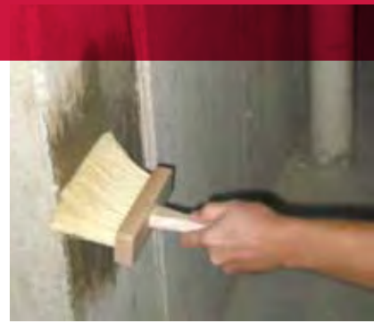
Applying waterproofing material with a masonry brush.
