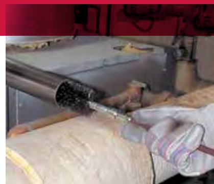
Cleaning boiler pipes with a flue brush.
