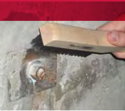
Removing excess concrete from the surface of a steel support plate.
