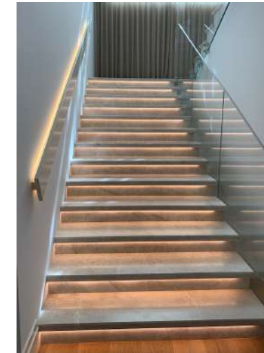
MARBLE STAIR WITH HIDDEN LIGHT
