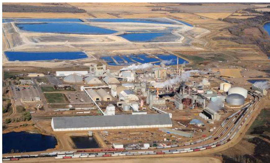
Photo 27. View of Agrium phosphate processing plant at Redwater, Alberta. The background shows phosphogypsum tailing ponds that possibly contain 70-85 % of rare earths originally present in phosphate ore. Source: http://www.miningandexploration.ca/alberta/article/albertas_industrial_heartland/
