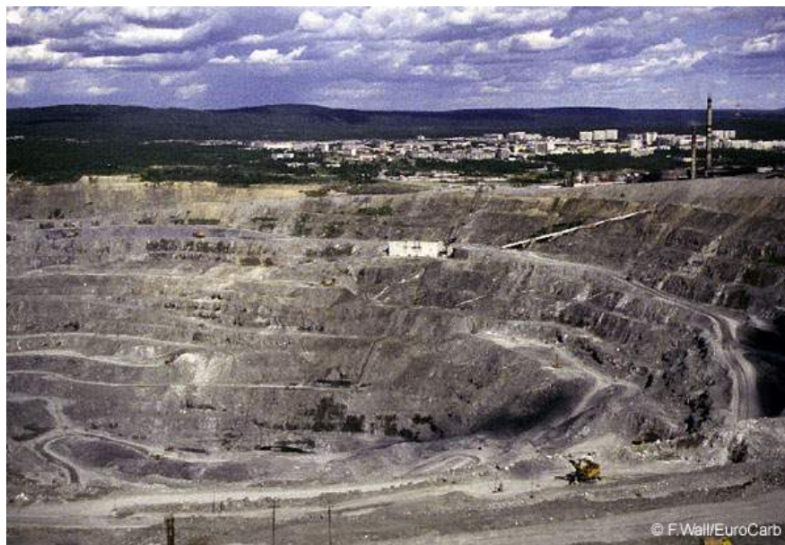
Photo 20. View of open pit at Kovdor phosphorite-carbonatite complex, Russia where numerous commodities are extracted: magnetite, apatite, phlogopite, vermiculite and baddeleyite: 512 mT Fe @ 25.4 wt.% ; 35 mT apatite rock @ 7.3 % P 2 O 5 ; 0.16 wt % ZrO 2 . The dark area comprises phosphorite cut by white carbonatite dykes. Photo by Francis Wall, University of Exeter.
