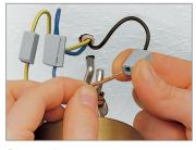
Removal: Squeeze connector housing and withdraw conductor
