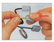
Removal: Hold wire to be removed and twist and pull the conductor
