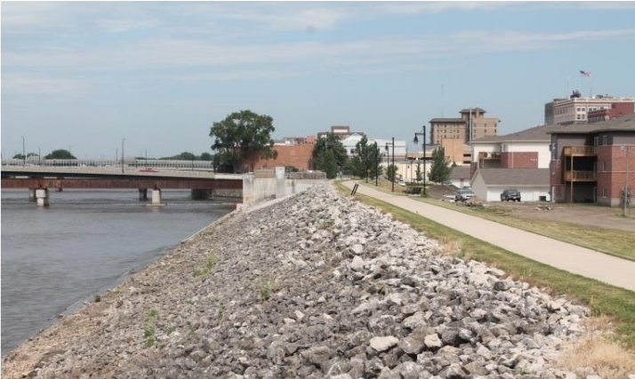
Flood levee prevents flooding of a town
