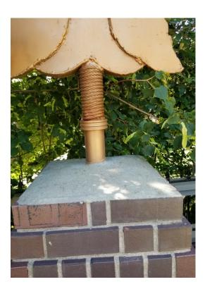
This arrowhead is from Wilson Street and is correctly mortared with a slope. However, the design is poor because the concrete cap does not overhang the brick column
