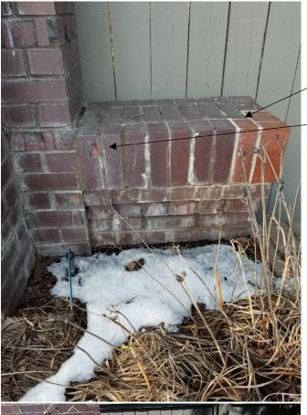
Replace these 4 bricks with salvaged brick. Install 1 16"x32" wall cap on top of wing wall.
