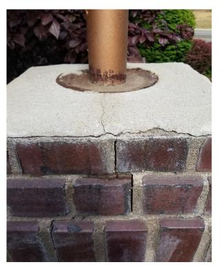
This arrowhead is from Center Street and is poorly installed in just about every way. The mortar cap allows water to enter the brick column from the uncovered metallic cup and through the crack in the mortar cap. This allows freezing water to enter the brick column and split the brick joints
