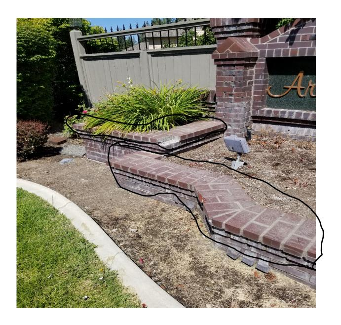
Remove top course of bricks from planters and salvage good brick for use in other areas with spalled or damaged brick.
