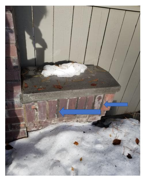
Unfortunately, this was not one of our ideal repairs. We wanted to replace the entire top row of vertical bricks but there just weren't enough good bricks left over. So, we simply capped the flat surface and re-pointed the mortar joints as best we could.
