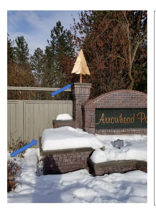
This is how our Center Street entrance looks after the repairs and with snow on top. Note that the caps all hang over the edge of the bricks. They do not drain onto other bricks.
