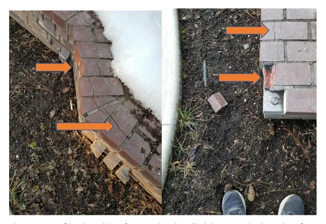
The top row of brickwork has fractured and spalled due to multiple cycles of freezing and thawing. Eventually pieces of brick simply fall off (called spalling).
