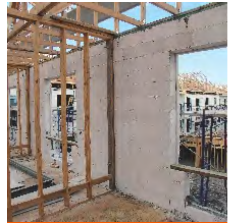
Fig. 21: Construction interior view.
