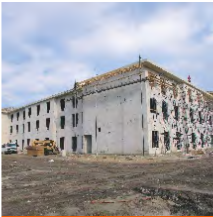
Fig. 22: Three-story hotel construction.
