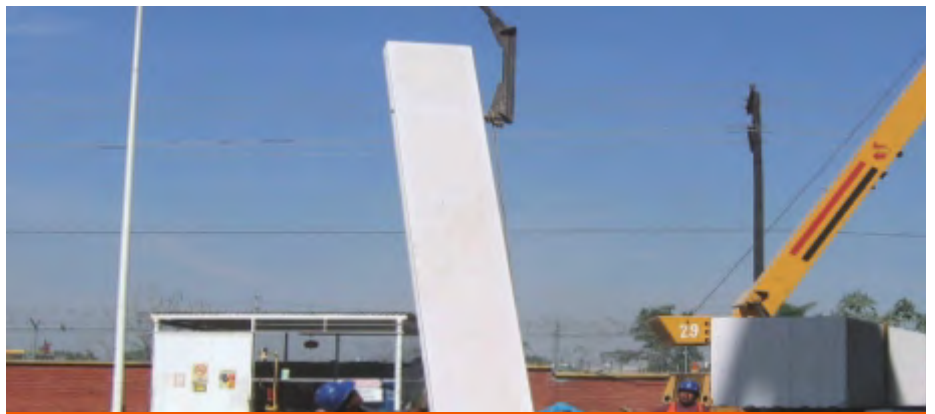
Fig.11: Place the lifting hook into the hole and lift the panel.
