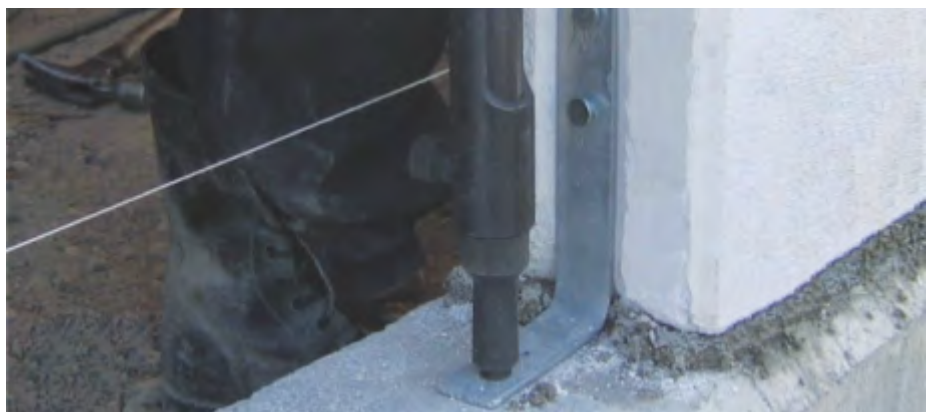
Fig.13: Fix the lower connector (type “B” connector).
