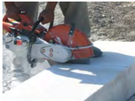
Fig.17: Cutting panel.
