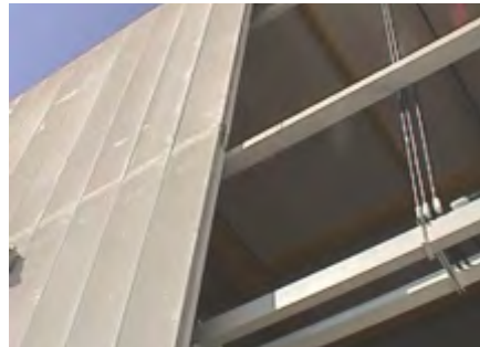
Fig.16: Second course of Hebel® Vertical Wall Panels.
