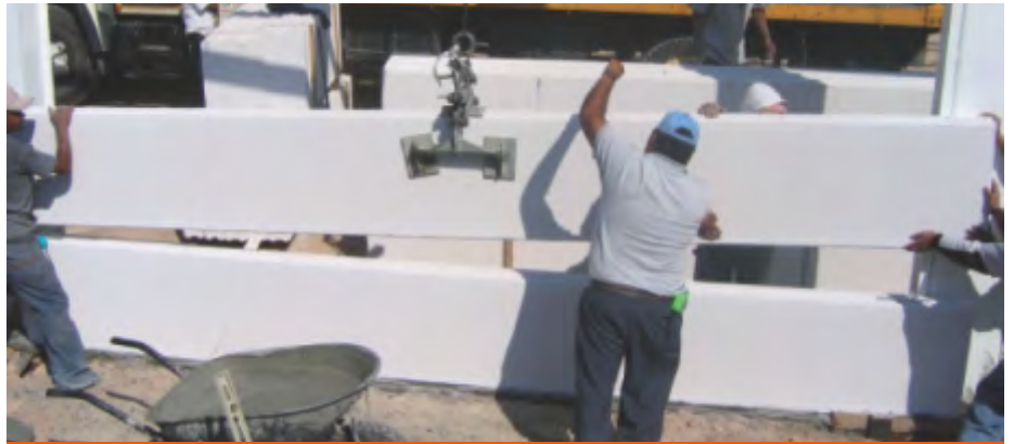
Fig.12: Once the panel in its position, check alignment.
