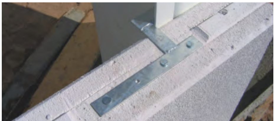
Fig.14: Typical upper connection (type “C” connector).
