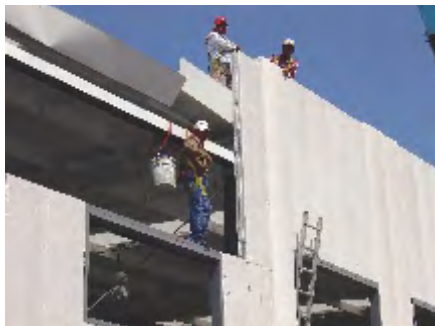
Fig.15: Plumbing the panel in second course.
