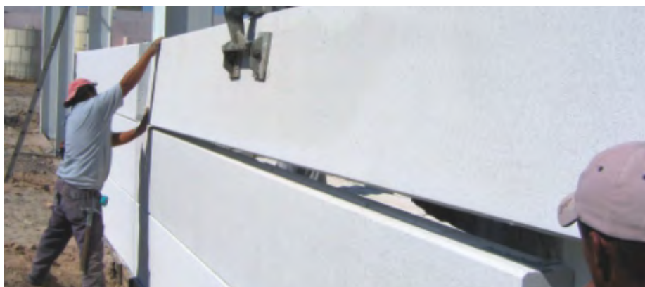
Fig.10: Stalling second panel.
