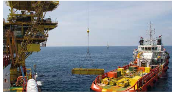
Offshore structure on open sea. Camera and monitor systems provide more precision in crane movements.
