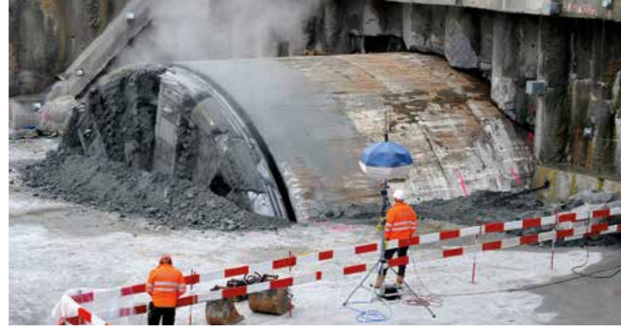
Tunnelling machine at work: Break-through of the drilling head with its rotating bits.
