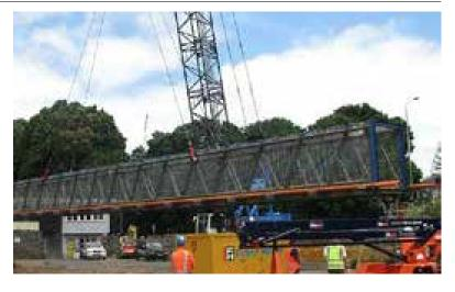
When possible, lower the working platform to the ground. Perform all work on a structure at ground level and then lift it into position once complete rather than taking the tools and equipment to height.  $\rightarrow$
