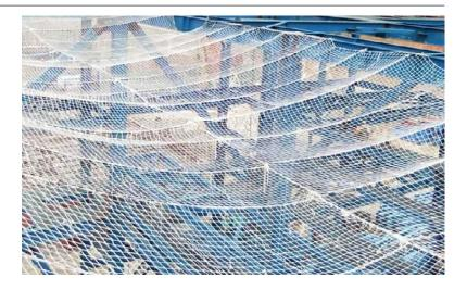
Utilise safety mesh or rated barrier netting (with debris lining) in areas outside walkways and underneath conveyors, walkways, platforms and along building/structure perimeters to prevent the drop of materials to a lower level.
