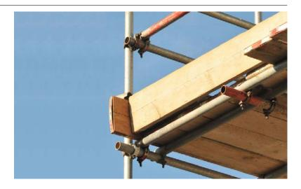
Toeboards and handrails should be fixed on scaffolding, platforms and walkways. By using additional closed mesh solutions, plywoods or other solid surface materials, coverage can be provided for all the gaps through which items can potentially fall.  $\rightarrow$
