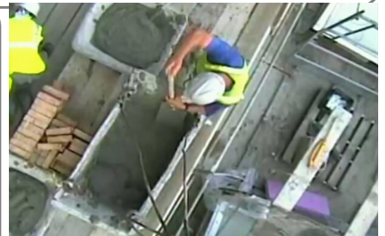
HoistCam™ Point of View Blind Lift Between Two Buildings
