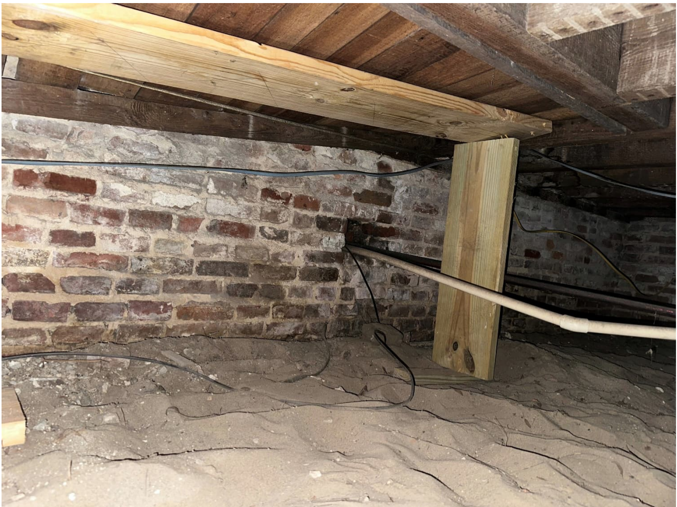
Photo #1 – View of Underside of Front Hearth
