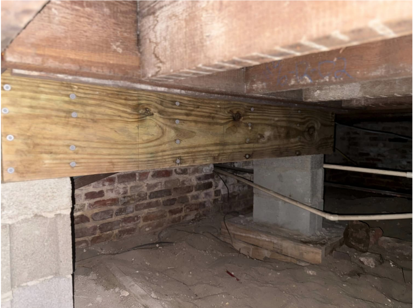
Photo #1 – View of New Support Beam, Piers and Footings
