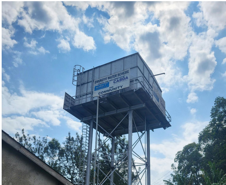
Figure 1 The Emukoye water-storage tower in Kakamega County. Visible infrastructure depends on governance, financing, technical capacity, and maintenance that continue long after construction.
