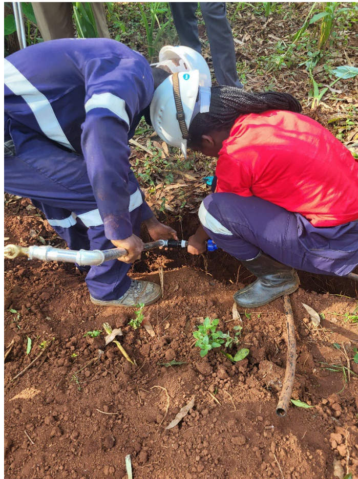
Figure 2 Local technicians connect distribution piping at Emukoye. Skilled installation is one part of the operational capacity required to sustain reliable water service.
