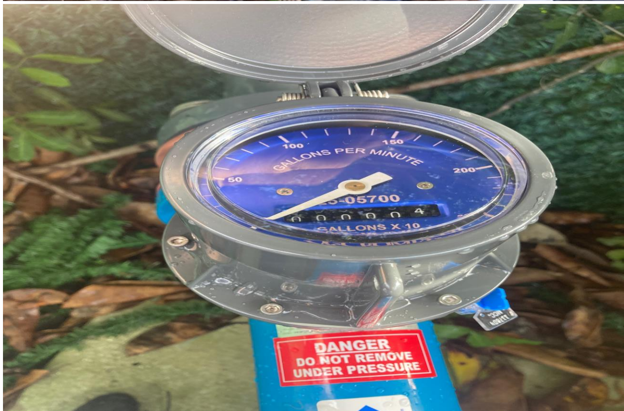
CAMDEN, SOMERSET SECTIONS. NEW IRRIGATION FLOWMETERS INSTALLED BY CHABOT IRRIGATION LAST WEEK.
