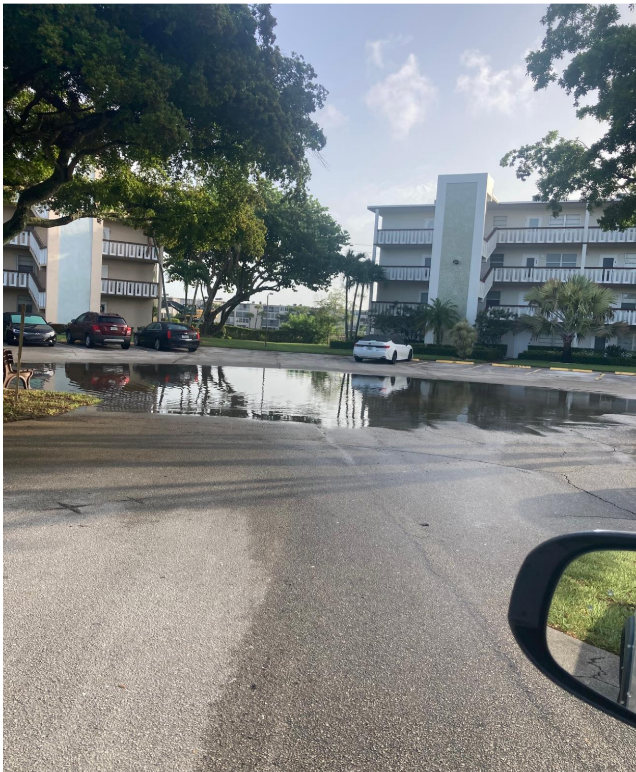
SOUTHAMPTON A/B- A STORM DRAIN CATCH BASIN AT THIS SPOT IS NON-FUNCTIONAL. DISCOVERED ON 6/28. ANCHOR MARINE WILL INVESTIGATE AND MAKE REPAIRS.
