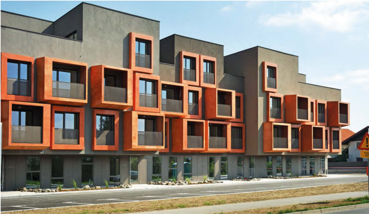
Jamaica Townhouse Apartment Project
