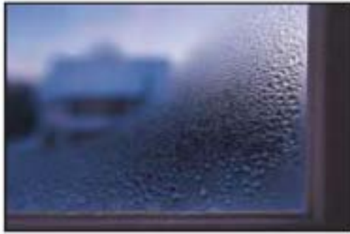
Condensation on the inside of a windowpane.
